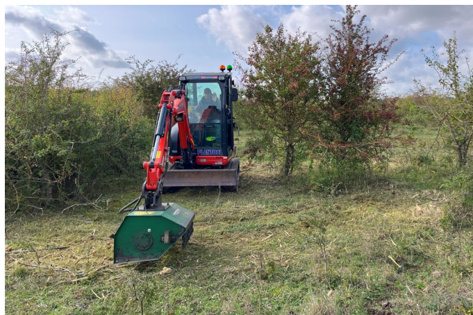
Spendlove Contracting sensitive scrub management in Shotley Quarry
